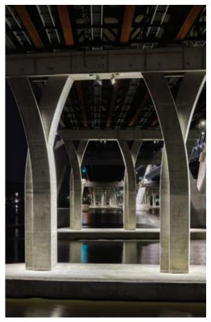
Dynamic uplighting brings the double—basket-handled arch structure to life at night. Color-changing luminaires focus on the bottom surfaces of the arches, creating an apex of color and light on this vital infrastructure project. Custom DMX controls were pre-programmed with dozens of celebratory scenes. They use slow movement and color shifts to provide visual interest without distracting drivers.
